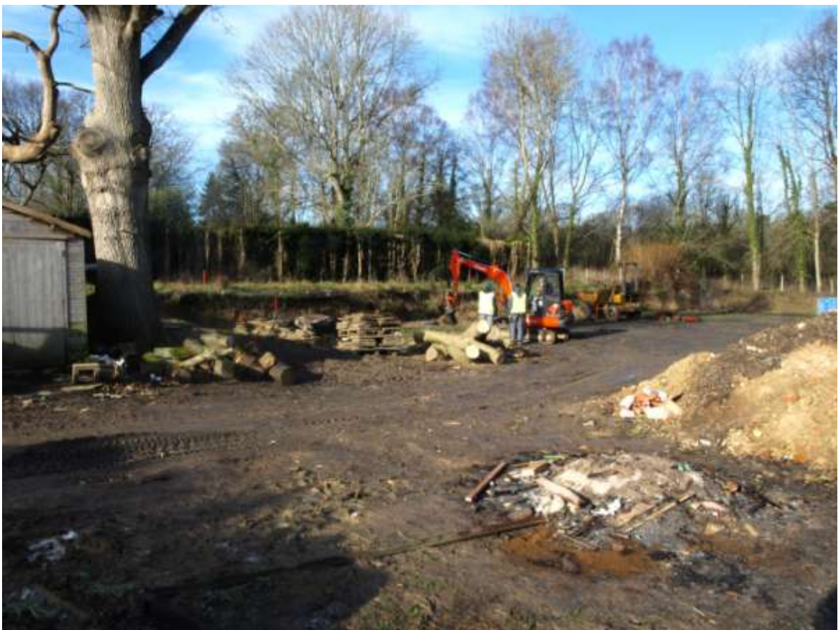
Plate 3: Looking North West at development site prior trench excavation.
