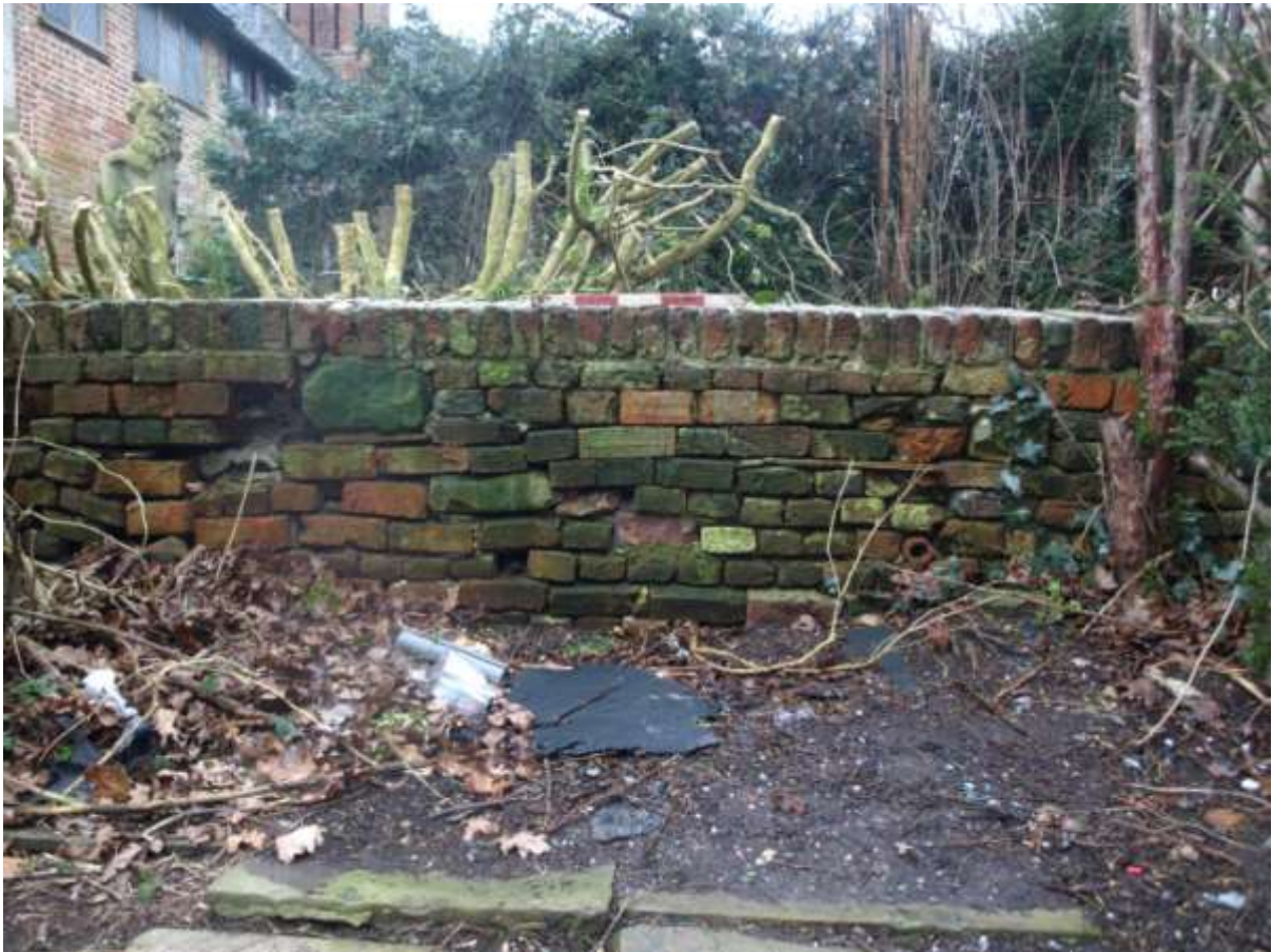
Plate 5: Looking west at wall [108]
