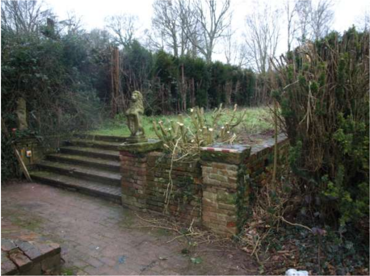
Plate 4: Looking North West at retaining wall [108].
